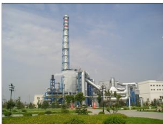
Source: China Energy Recovery
